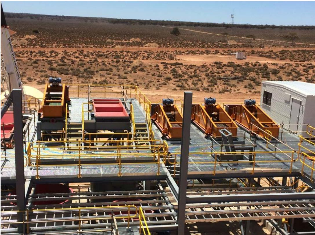
Figure 3 | Underflow hoppers and screen decks being installed
