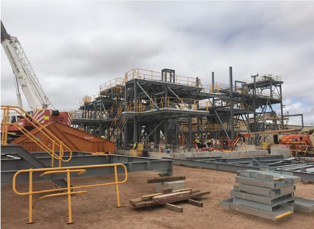
Figure 2 | Structural steel – main DMS building
