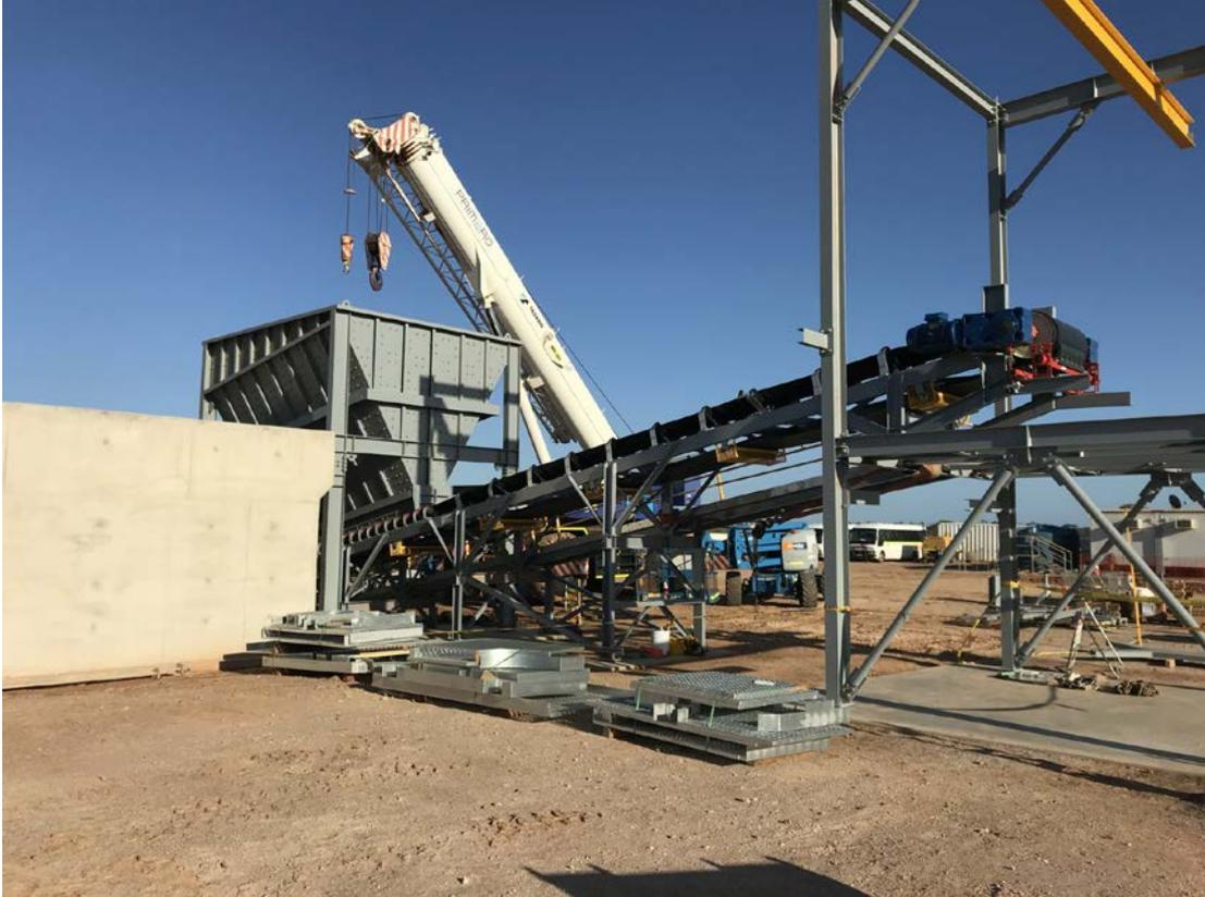
Figure 6 | ROM Feed Bin and Transfer Station
